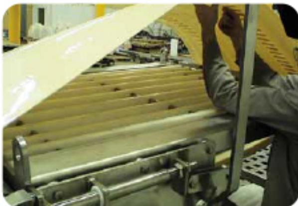
Belt repaired on site.
